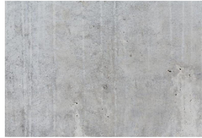
GREY MATTE STAINED/SEALED CONCRETE
