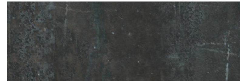
BLACKENED SHEET STEEL @ WALLS + C.TOP SUPPORTS
